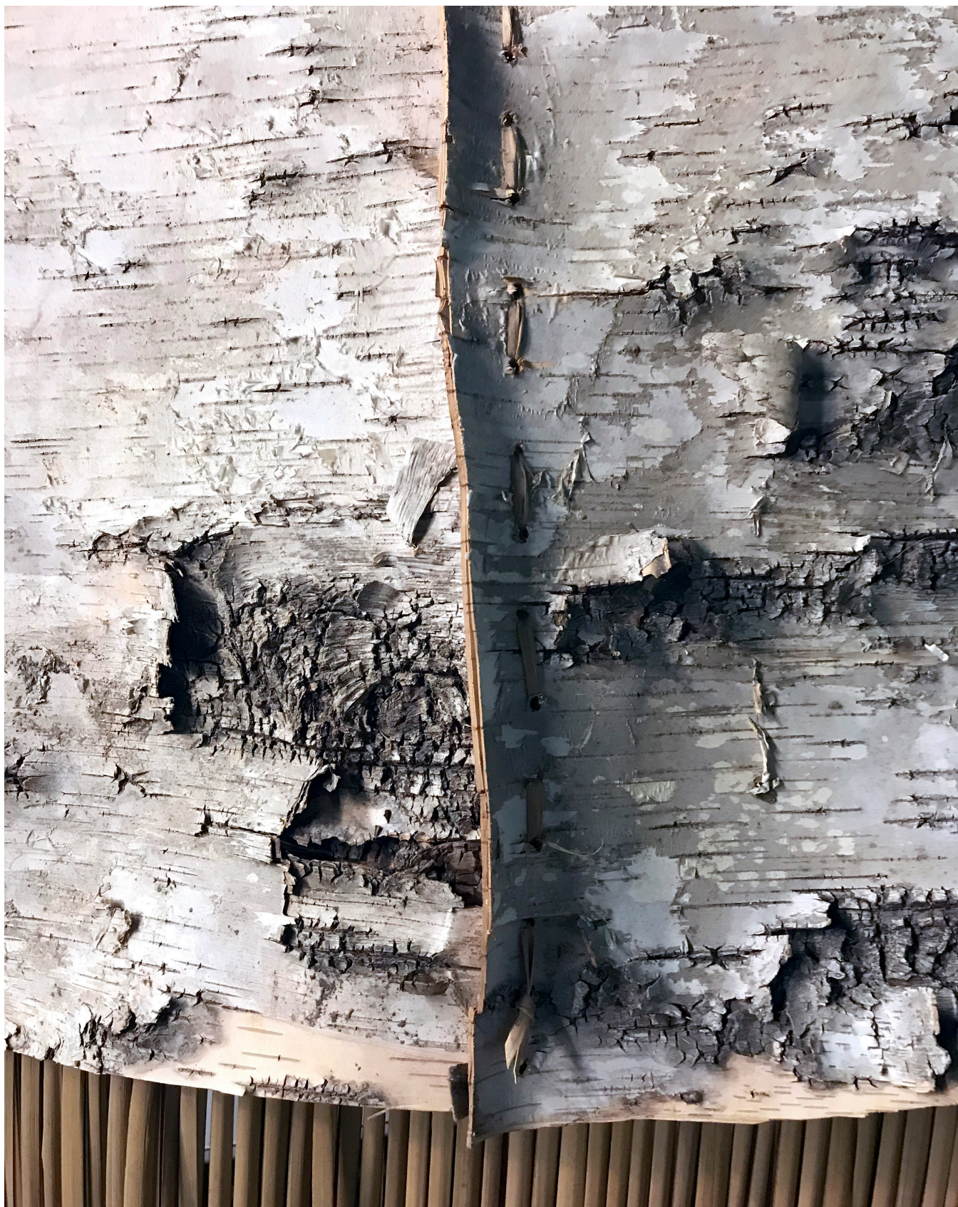
Figure 4. Wiigwaasibakoon and reed mat insulation on a waaginogaan . Author's photograph at Ziibiwing Center of Anishinabe Culture & Lifeways.
